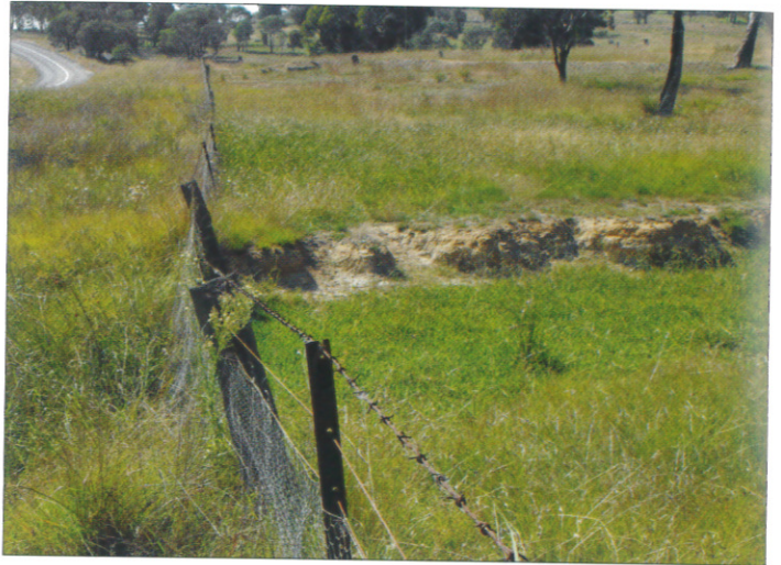
We see small erosion cuts like this so often that we hardly notice them. They are evidence of a degraded water cycle and we need to fix them.
