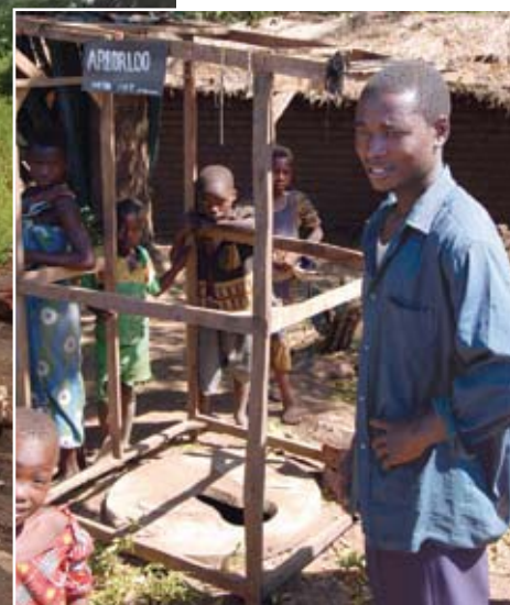
Construction of an arbor loo.
