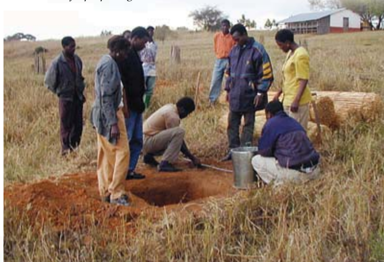
Construction of an arbor loo.
